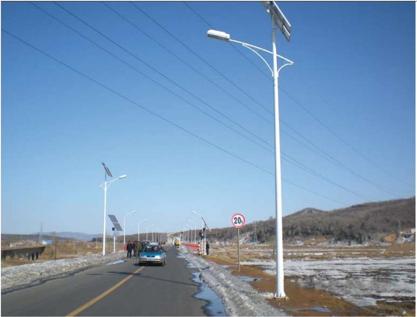
The municipal government of the Heilongjiang province in China installed 232 solar street lights equipped with Phocos CIS charge controllers along the 9.2-kilometer road to the airport in the Hegang district of Xing'an.
